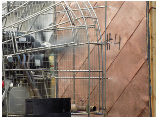
Figure 15.6.3: Diagonal copper flat lock cladding tested by the AAMA 501.1 dynamic pressure water penetration procedure.
