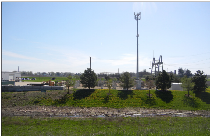
Figure 1. One of Involta-Marion's two utility feeds is literally next door. The second primary feed originates at another substation about five miles away. Redundant utility feeds are a primary requirement for Tier III compliance.
