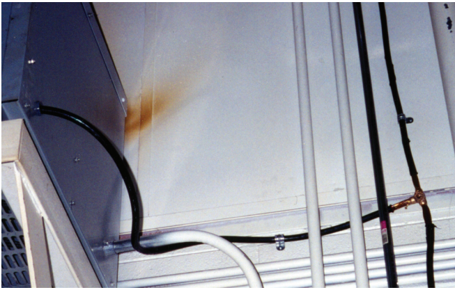
An overhead-mounted 480/240V CNC equipment transformer properly connected to the building's grounding system using #4/0 AWG copper, which is larger cable than that required by the NEC. The vertical ground conductor at far right is bonded to the building steel (not shown), which PowerEdge Technologies used as the building's reference grid.
