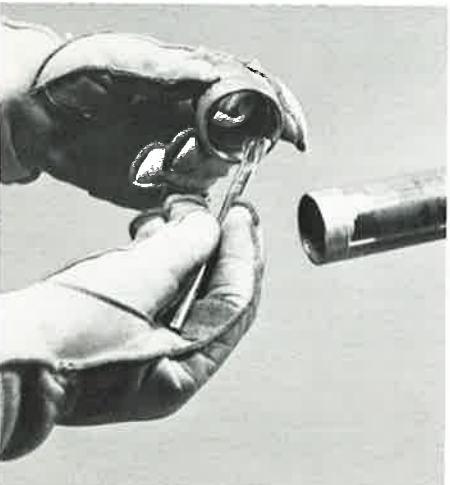
FIGURE 8. FLUXING THE FITTING
