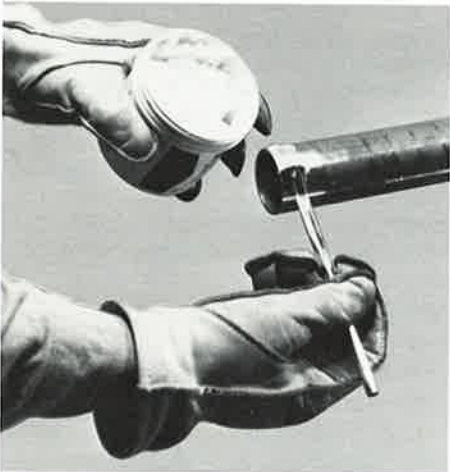
FIGURE 7. FLUXING THE PIPE
