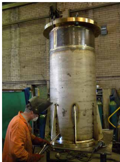
Figure 56 - Low temperature pre-heating of weld bead prior to second run (Courtesy Bailey Manufacturing, Stoke-on-Trent, UK)
