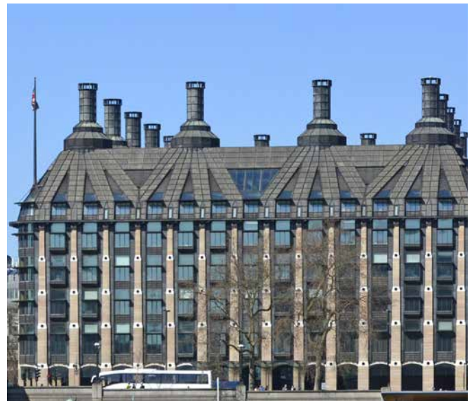
Figure 4 – Nickel aluminium bronze roof, Portcullis House
