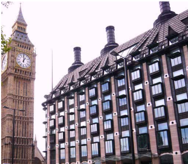
Figure 3 – Nickel aluminium bronze window frames, Portcullis House
