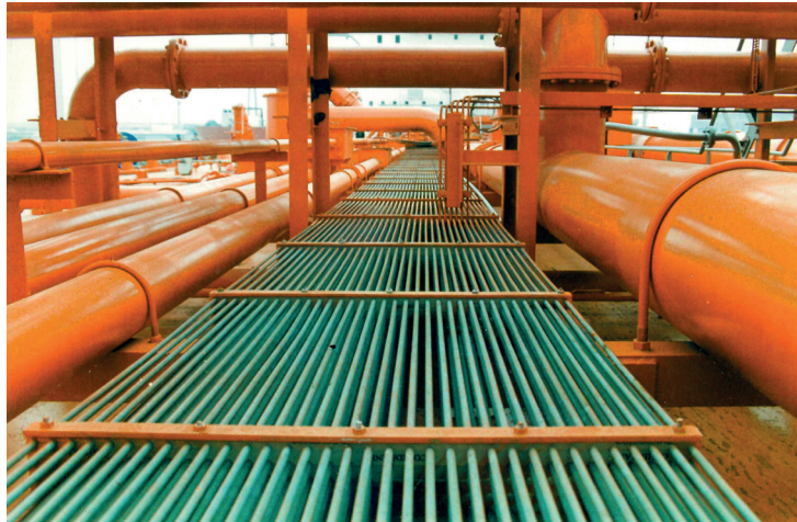
Figure 1 - 90/10 copper-nickel piping on a marine chemical tanker (Courtesy of Eucaro Buntmetall)
