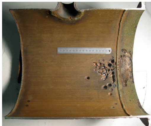
Figure 6 - Pitting attack of 90/10 copper-nickel due to sulphide in the seawater (Courtesy of Intertek)
